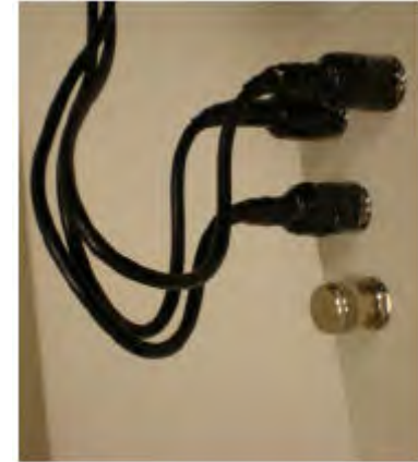
FIGURE 21 Creating Cable Drip Loops
