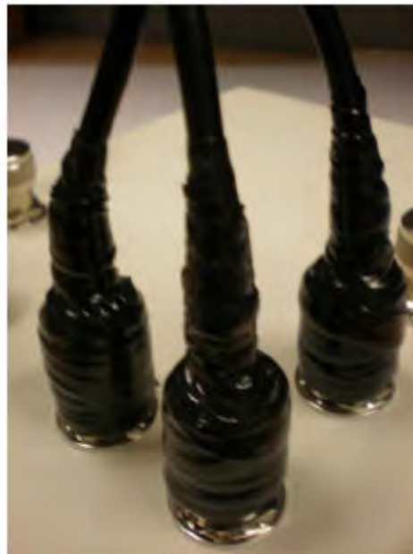
FIGURE 20 Repeating for Other Cables
