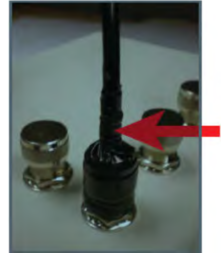
FIGURE 15 Wrapping the Electrical Tape
