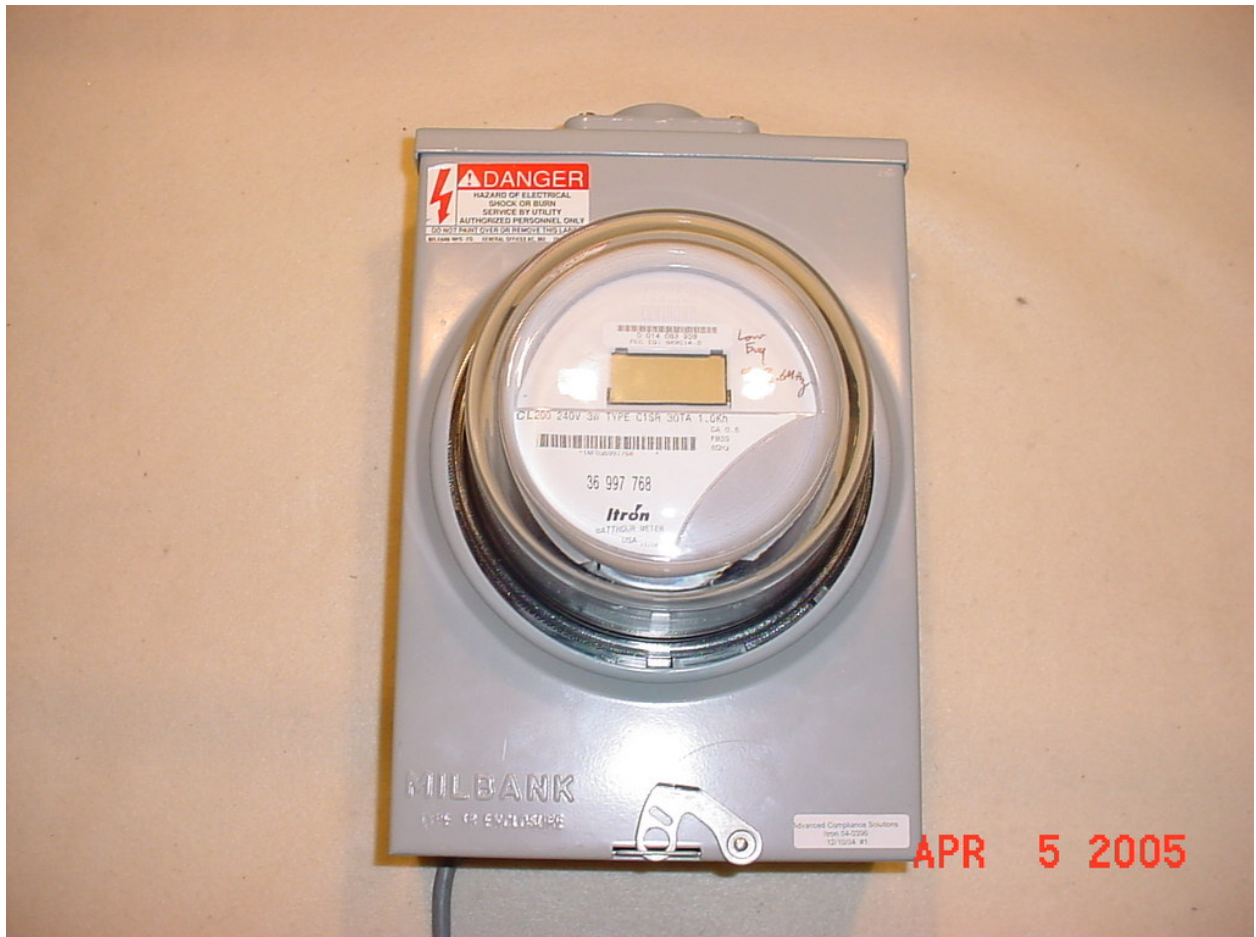
Figure 1: External – Front View
