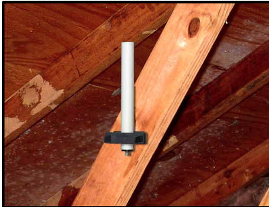
Figure 7 - Secure Signal Antenna to bracket
