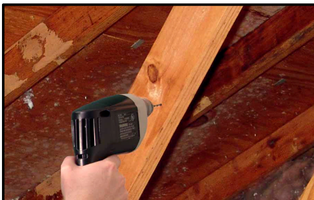
Figure 5 - Drill two holes for mounting bracket
