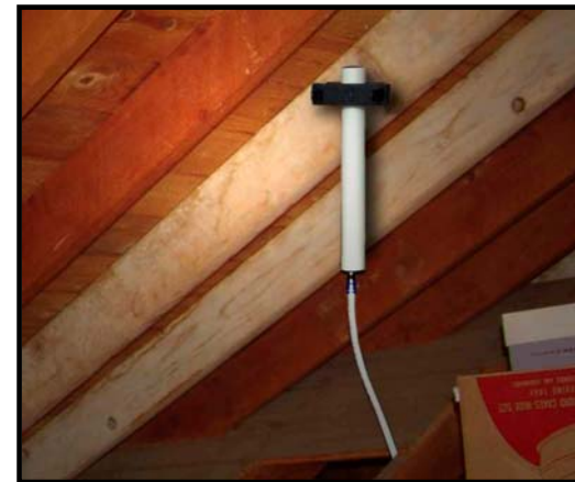
Figure 5 - Mounting Signal Antenna to a Main Beam
