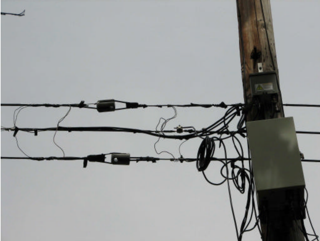
Installation of the overhead capacitive coupler on the LV line
