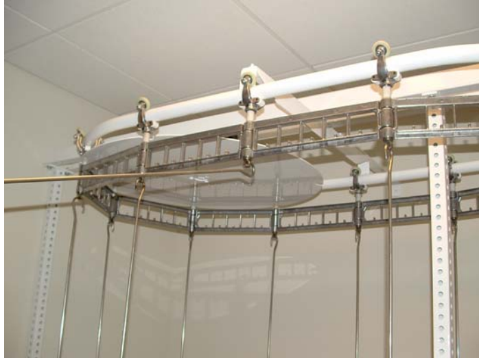
View of drop rods being attached to the Wardrobe valet
