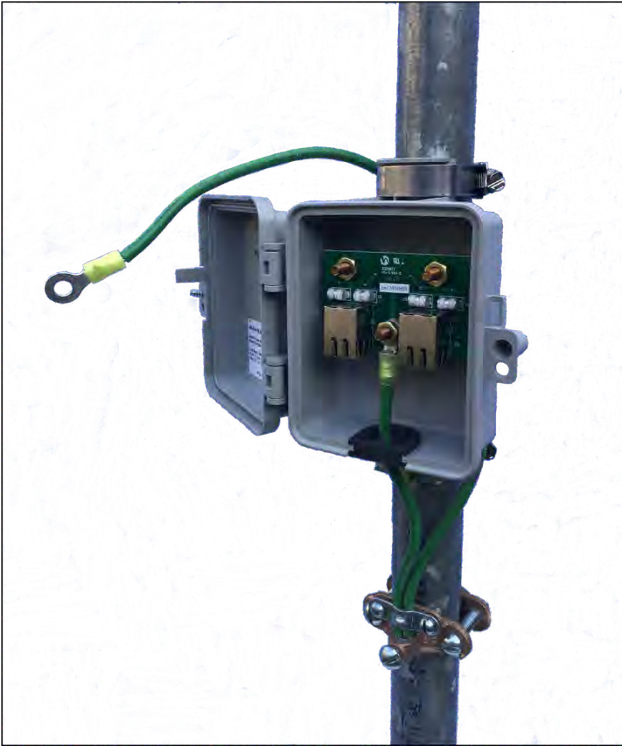
Figure 17: Attach the ground wire
