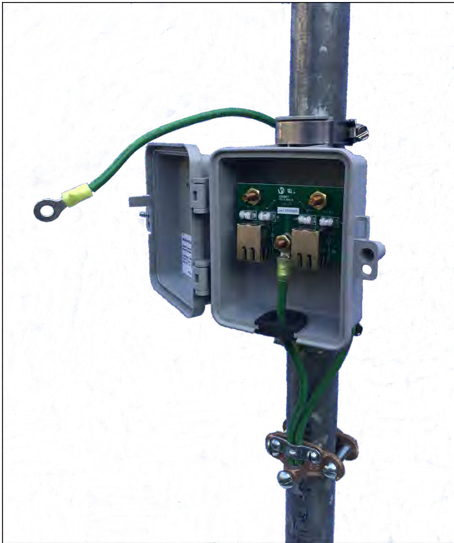
Figure 17: Attach the ground wire
