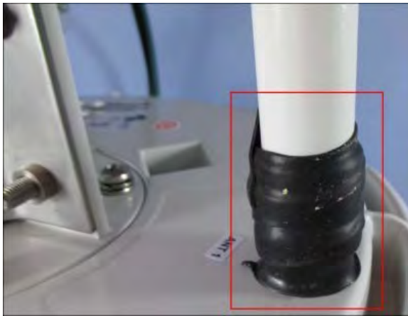
Figure 40: Layer of rubber insulation on antenna connection
