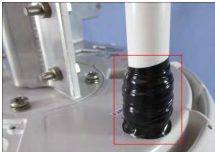
Figure 41: Outer layer of tape on antenna connection
