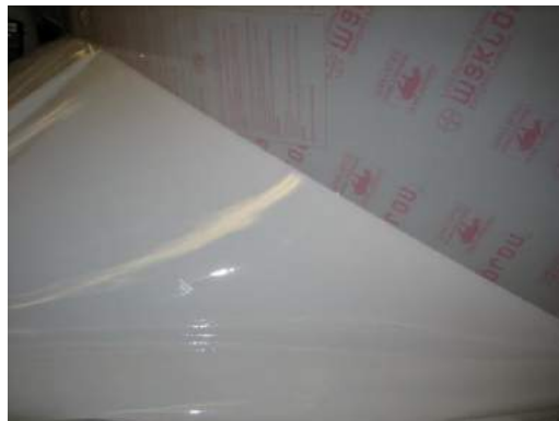
Figure 63: Scratch Guard Film Being Removed
