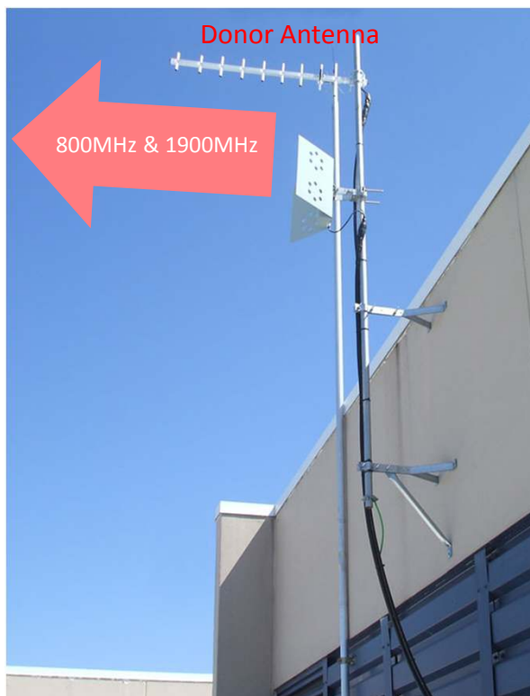
Existing Donor Antenna for both 800MHz and 1900MHz
