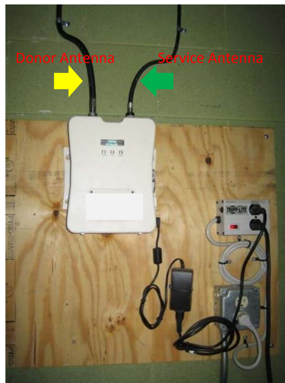
Existing Donor Antenna for both 800MHz and 1900MHz
