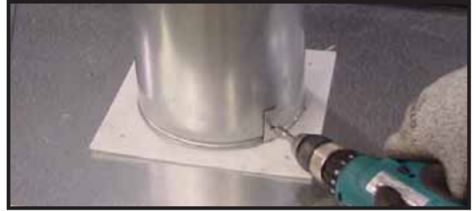
Figure 9.3 Gasket in Place
