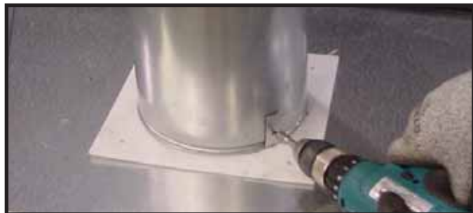
Figure 9.3 Gasket in Place
