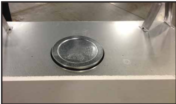
Figure 9.1 Seal Cap in Position
