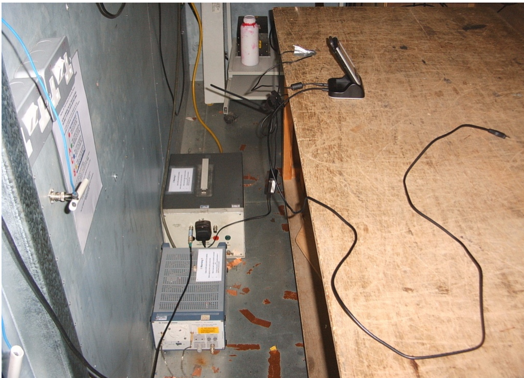
Photograph 2 Conducted Emissions - Back
