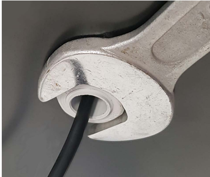
Figure B-10 - Secure Cable Gland with Nut
