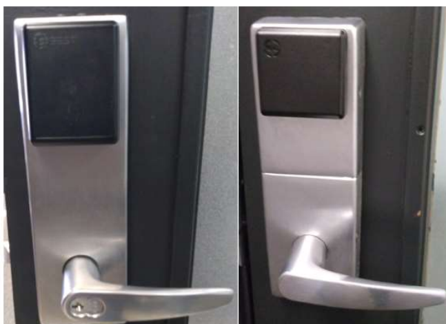
Inside escutcheon (antenna location)
