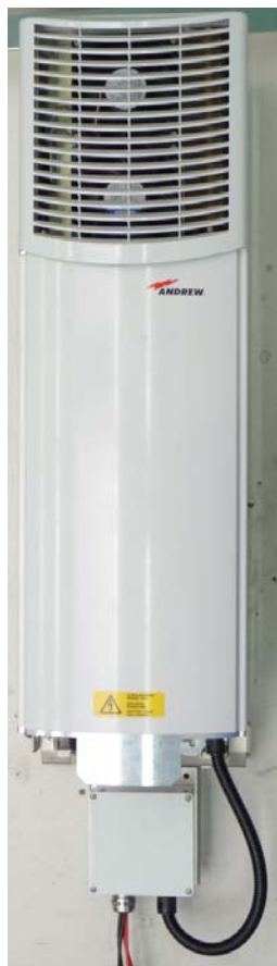
figure 3-8 Mounting of DC Box, finished
