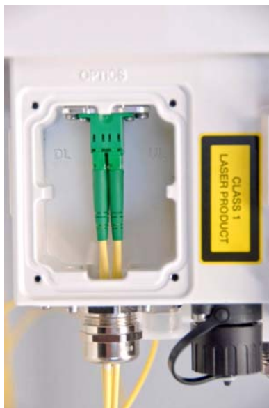
Figure 2-23 Optical cable installed
