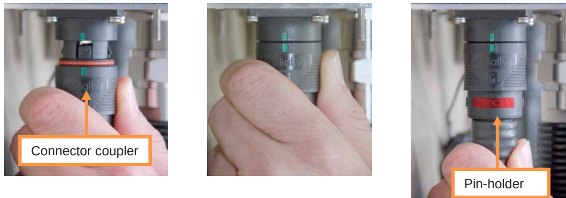
figure 4-19 Mounting the EU cable bridge
