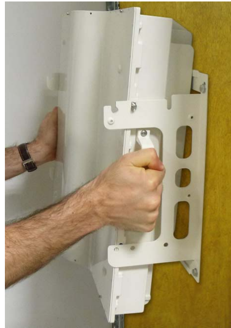
figure 4-10 1 st unit placed on wall mounting bracket
