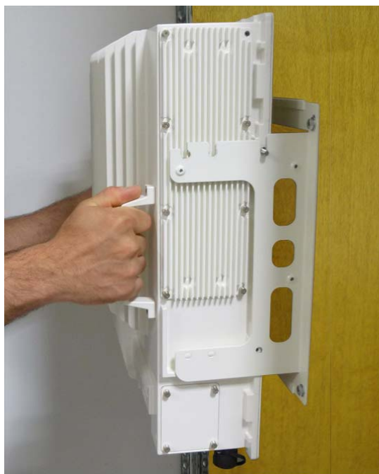
figure 4-6 Place EU onto wall mounting bracket – single mount
