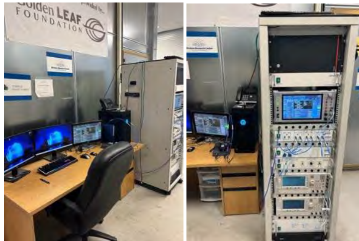
Figure 2 WRC workstation and Chamber Equipment
