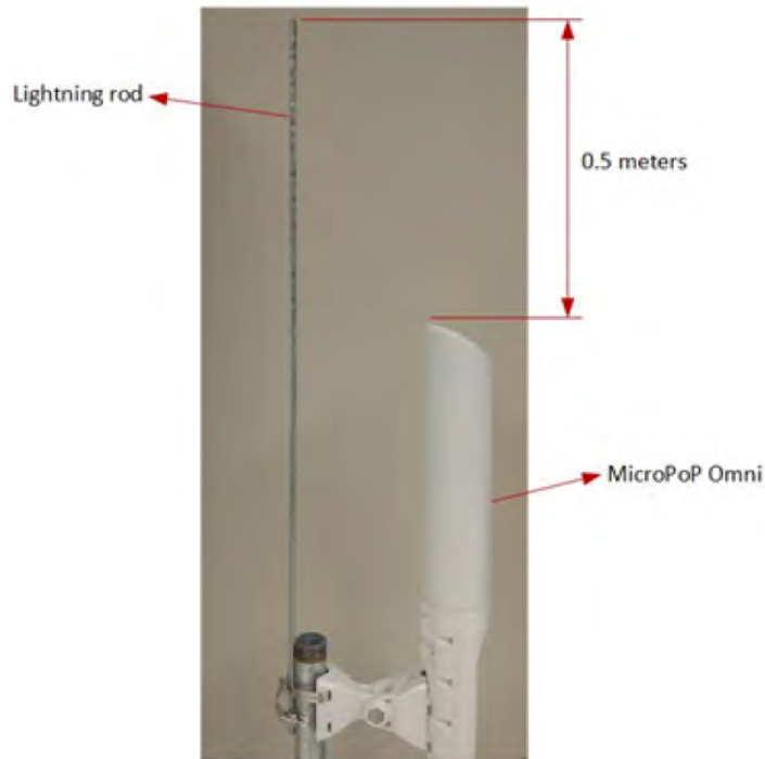
Figure 40: MicroPoP Omni with Lightning rod
