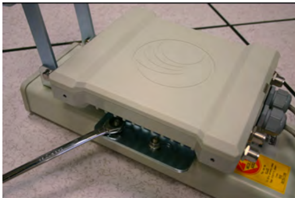
Figure 137: Lower bracket attached to AP antenna
