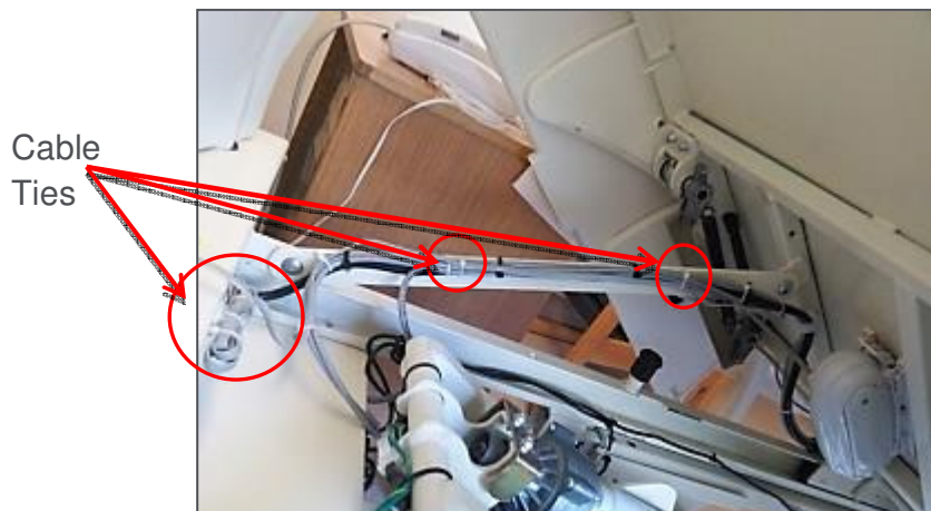
Figure 5. AC Line Power Sensor Cable Routing
