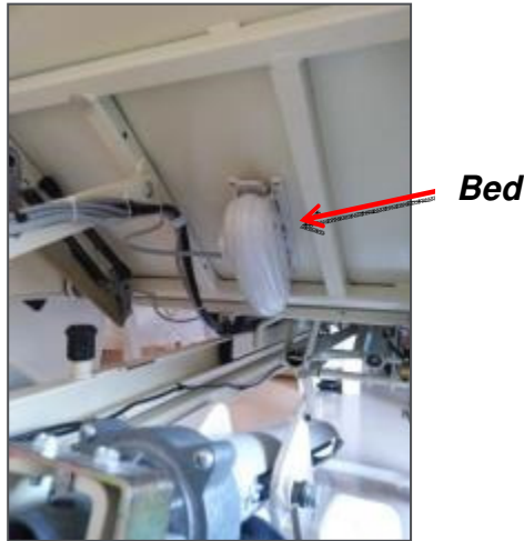
Figure 1. Bed Beacon Installation Location
