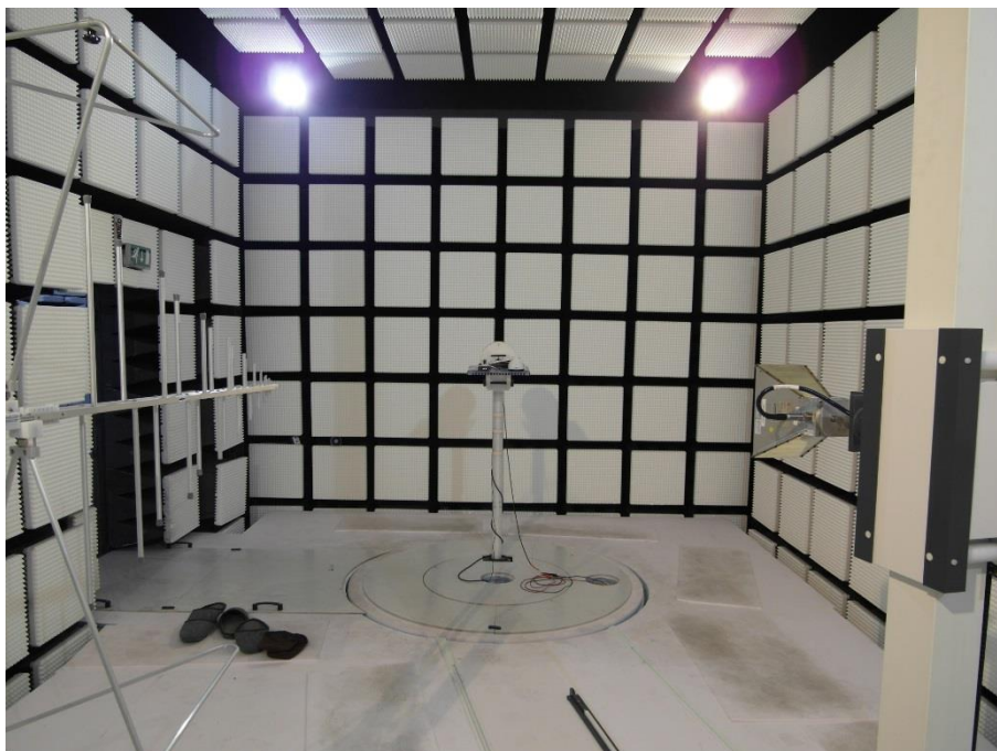
Photo 6: Fully Anechoic Chamber
