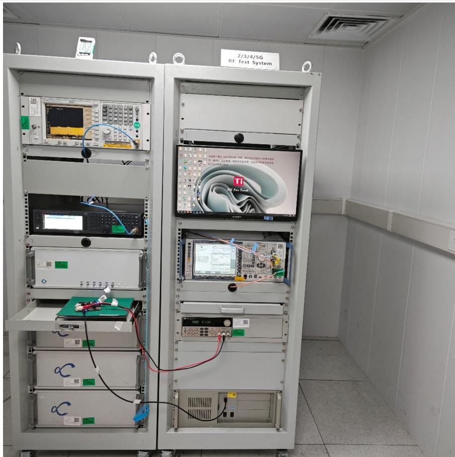
Conducted Test- RF
