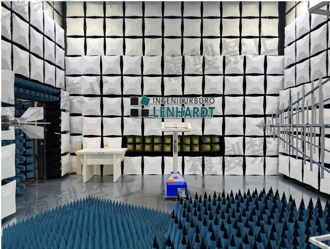
Photograph 30: Radiated measurement, overall view.
