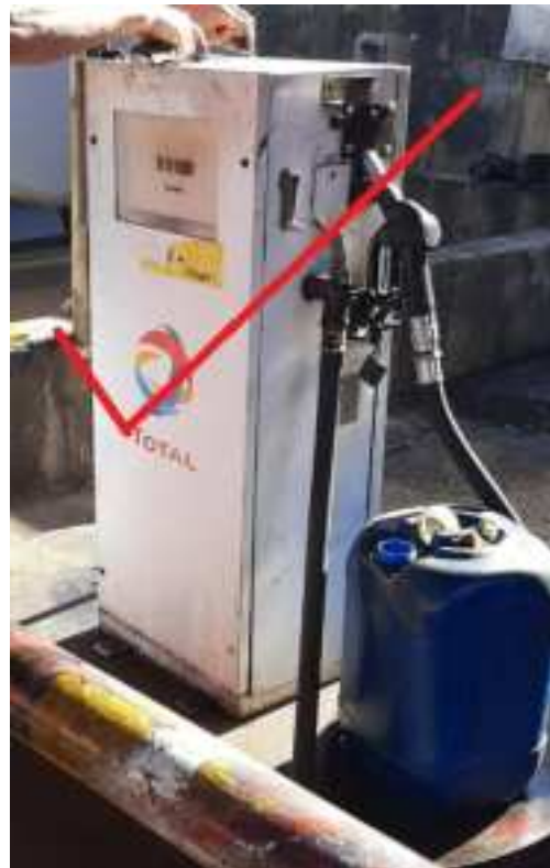
A perfect covert installation.
