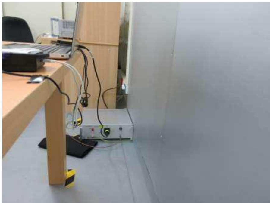
Photograph 8: Set-up for AC Mains (Back View)
